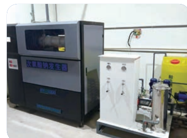
Xinjiang Aketau Water Treatment Plant Project
