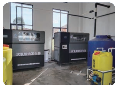
Heyuan Water Plant Project, Guangdong
