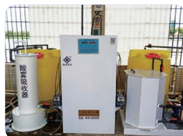
Fujian Longyan New Rural Drinking Water Project
