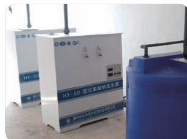
Xining New Rural Drinking Water Project, Qinghai
