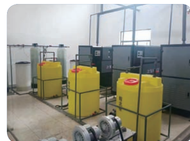
Jiangsu Yangzhou Water Treatment Plant Project
